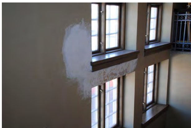
Photo 4 and IR photo 5. A severe damage at the first floor have appeared and the low surface temperatures is giving f = 0.71 just above the limit of risk for condensation and mould growth in the construction. Photo to the left by Maja Lindman and to the right by Heidi Norrström.
