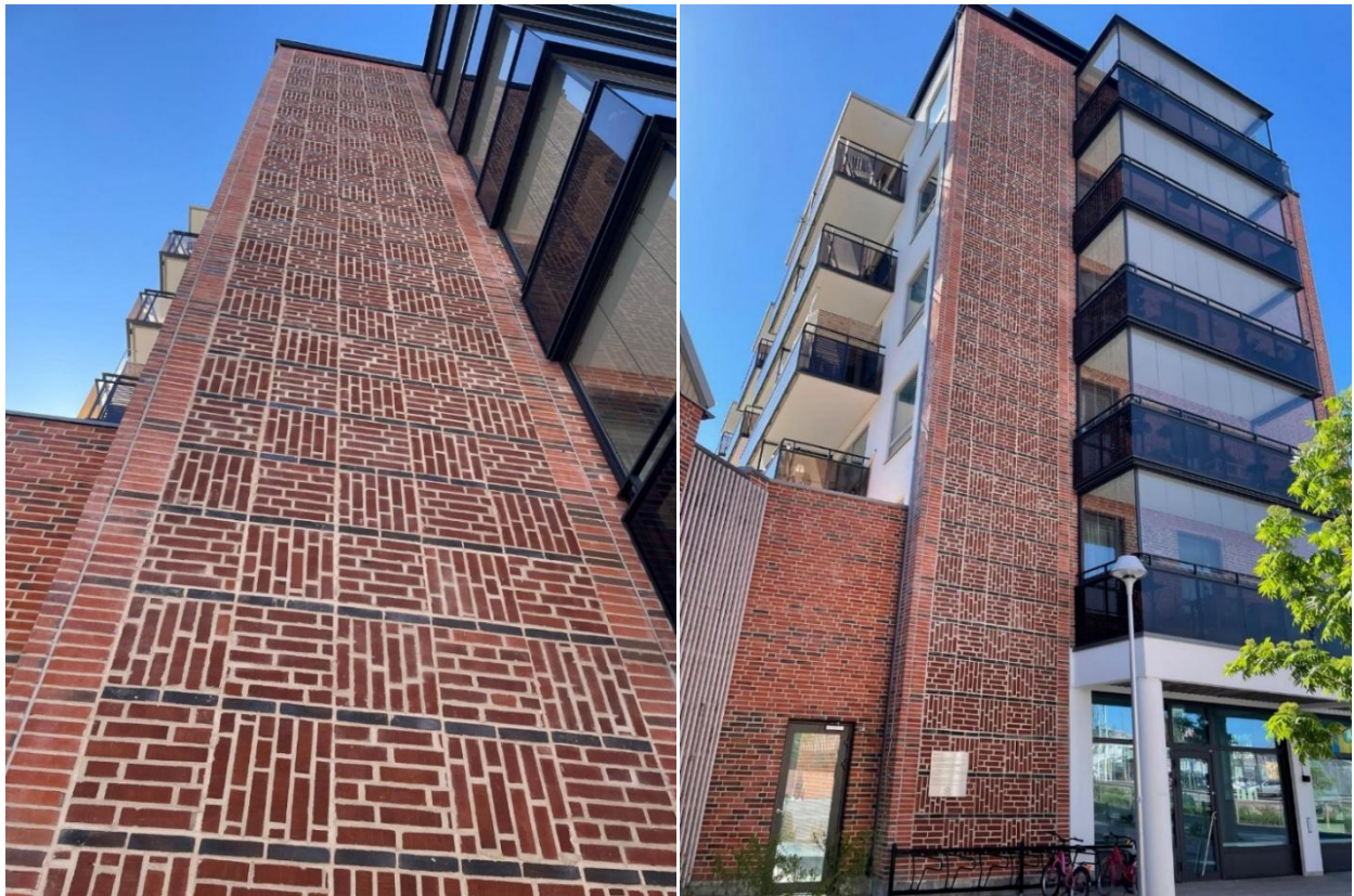
Figure 13: The recycled bricks are used as façade bricks in the new façades in Drottninghög, Helsingborg
