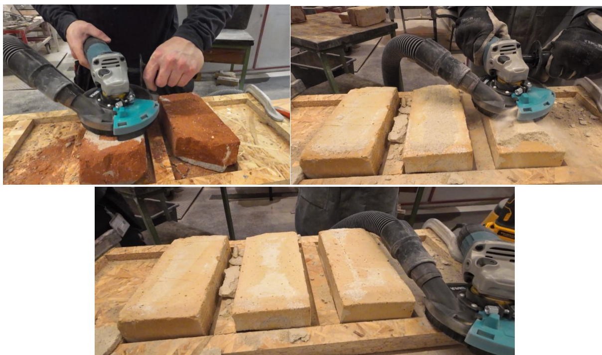
Figure 11: Cleaning of the bricks by angle grinder technique (taken by Rasmus Stenholt-Jacobsen)
