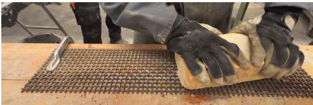
Figure 5: Cleaning of the brick by friction and raking on steel mesh (taken by Rasmus Stenholt-Jacobsen)
