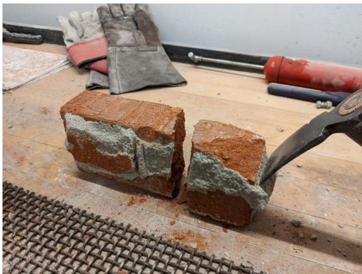
Figure 10: Cleaning of the brick by chisel hammers (taken by Rasmus Stenholt-Jacobsen)
