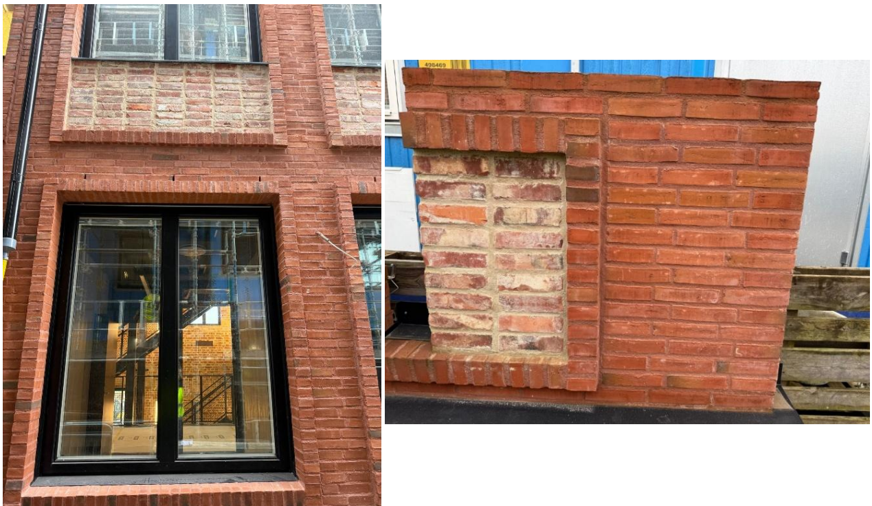
Figure 14: Façades built with a mix of new and recycled bricks in Spritfabriken in Eslöv (taken by Mohammad Kahangi)
