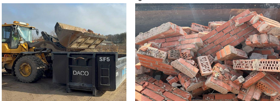
Figure 3. Reclaimed bricks collected after demolition are to be delivered to Brukspecialisten
