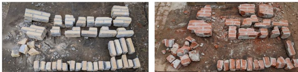
Figure 7. Different steps were taken to assess the separability, showcasing the demolition practice in reality – Number of full and half bricks salvaged after separation and demolition
