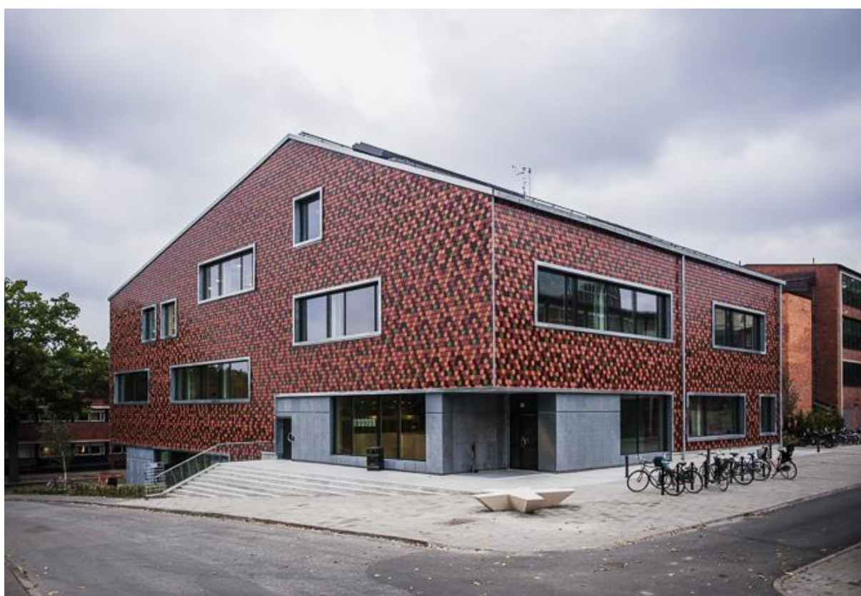
Figure 48 Testbed AH in the KTH main campus in Stockholm 1 .
